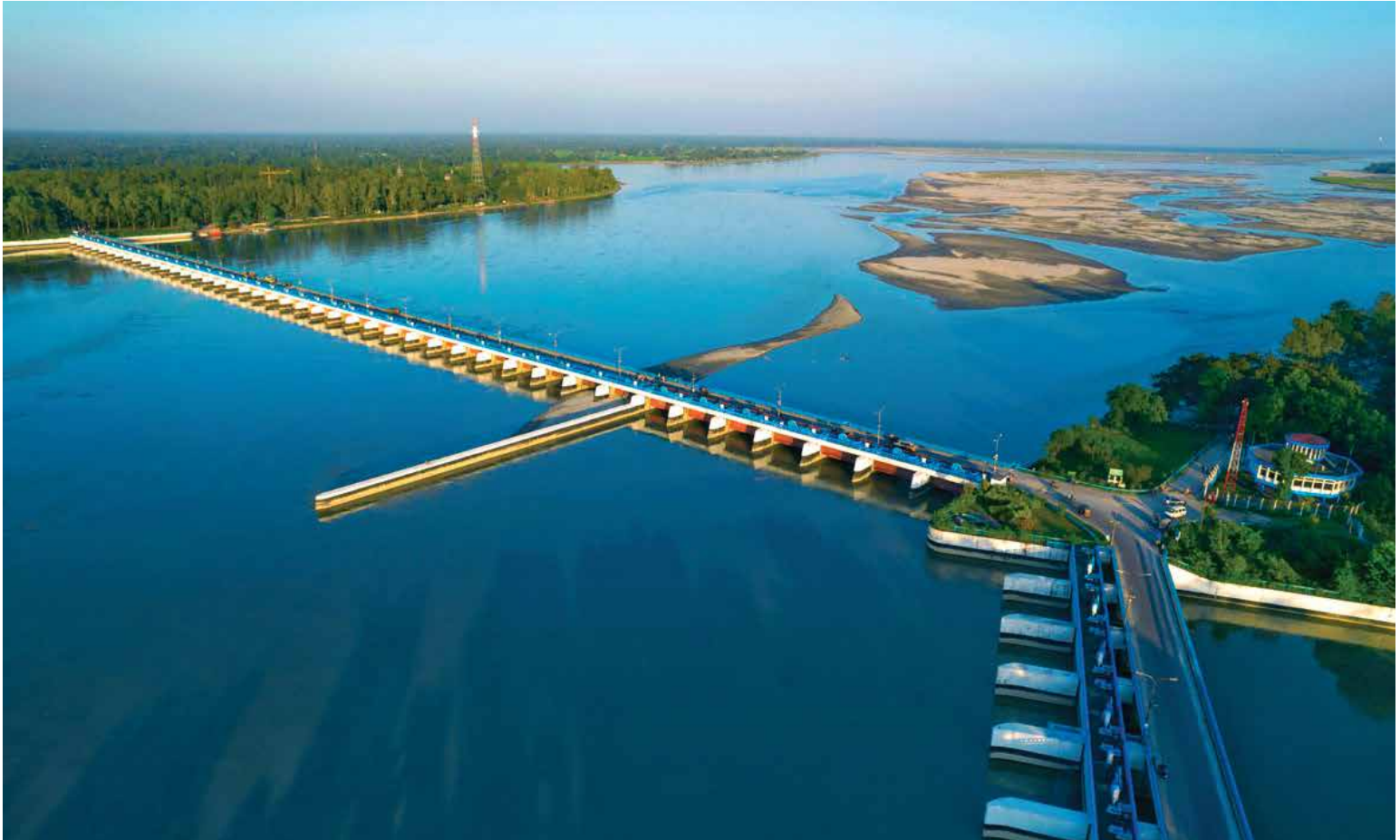
The Teesta Barrage Project is the largest irrigation project of Bangladesh. It stands across the Teesta river at Dalia-Doani point in Lalmonirhat district. The project is bounded by the Teesta river on the North, the Atrai river on the West, Shantahar-Bogra railway line on the south and Bogra-Kaunia railway line on the East. The project covers seven districts of northern Bangladesh. Photo : Md. Shafiu Islam Shaikot
