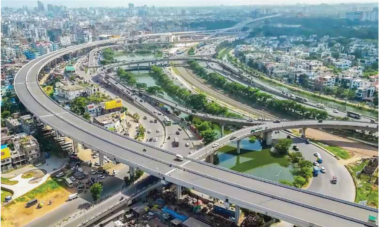
Kuril Flyover and Expressway. Dhaka. Photo : Press Information Department, Bangladesh (PID).
